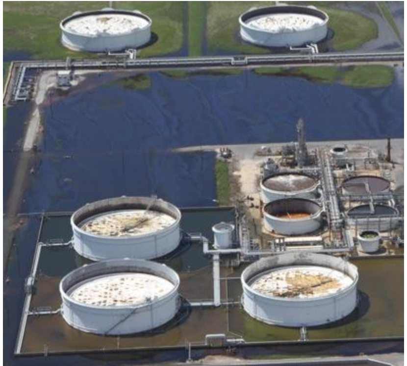
Oily sheen on water at the flooded Phillips 66 Alliance refinery in Belle Chasse observed by a GMC overflight on September 2.
